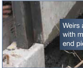
Weirs are constructed with male and female end pieces.
