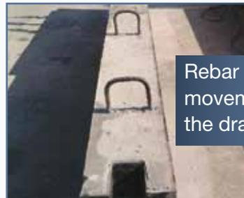
Rebar allows for easy movement of weirs in the drainage ditch.
