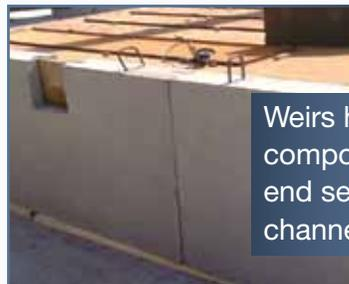
Weirs have two components: 4-foot end sections and 6-foot channel sections.
