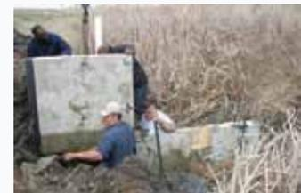
Ensure the sections are tightly locked. There will be some space between sections that will fill with sediment and rust over time.
