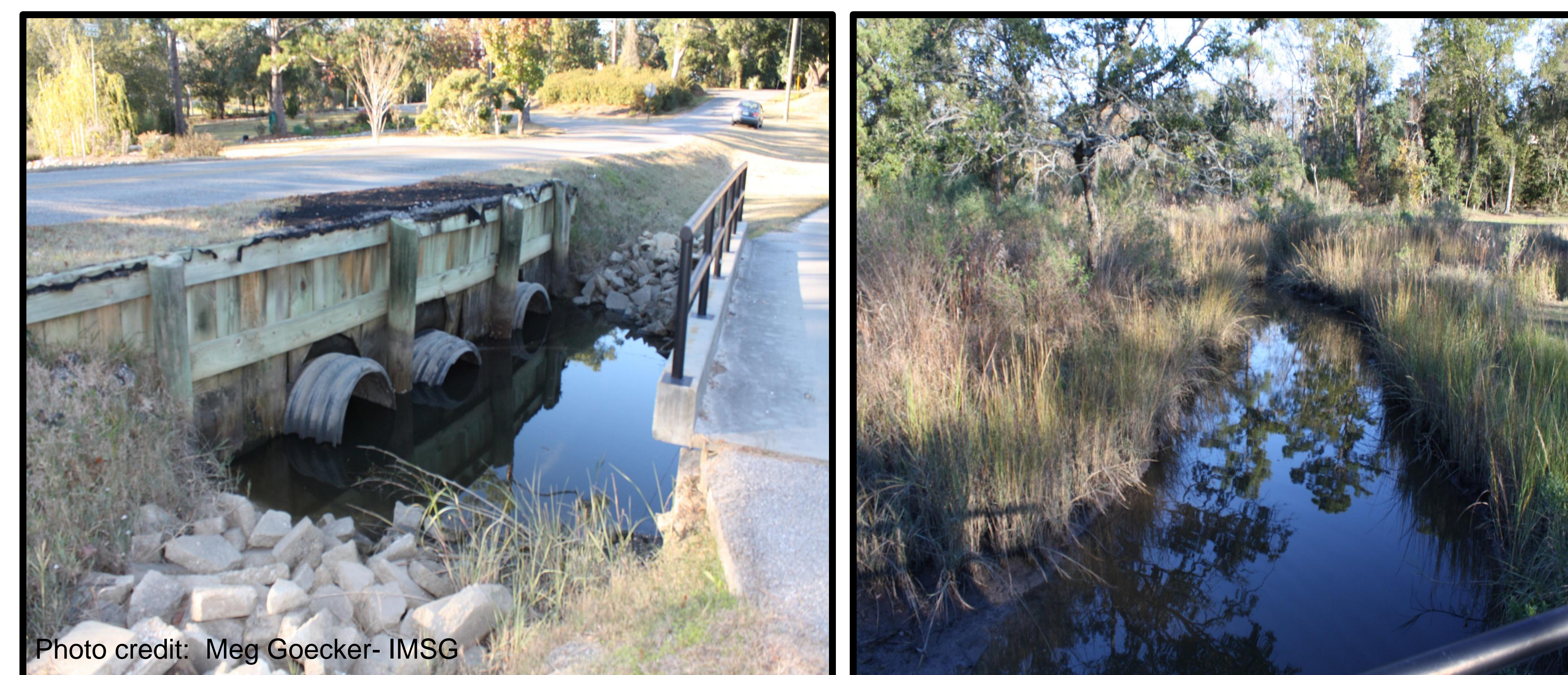
Figure 3. Undersized culvert (barrier) and the habitat (impact area) behind the barrier that would benefit from increased tidal flow as identified in Figure 2.
