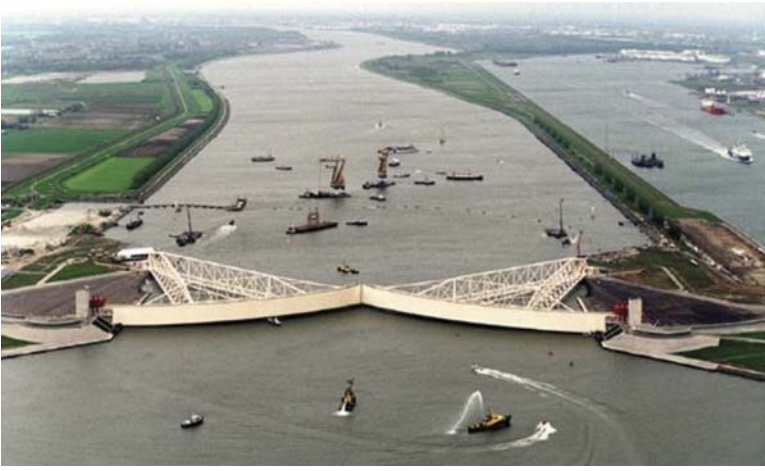
This retractable storm surge barrier spans 3,000 meters across the Eastern Scheldt in the Netherlands. ANP-Foto
