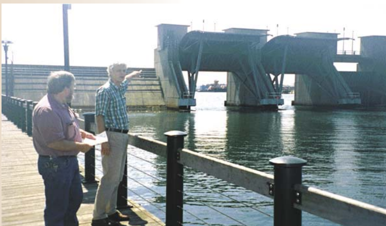
Co-investigators Roger Flood (l.) and Robert Wilson (r.) view the three Tainter gates at the Fox Point Hurricane Barrier in Providence, RI. Others working with the research group are Douglas Hill, Brian Colle, Frank Buonaiuto and several students. Photo by Douglas Hill
