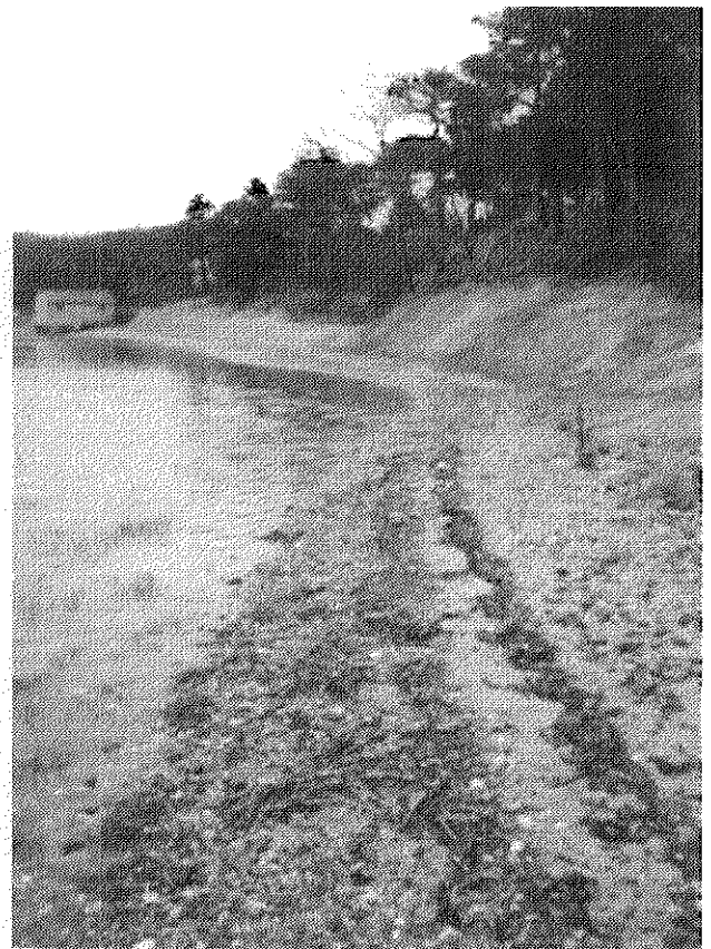
Fig 34. Bournes Pond bank stabilization project completed
