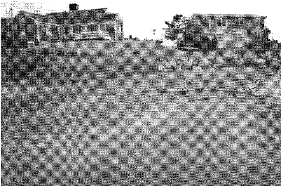
Fig 36. Using fiber rolls to construct a return
