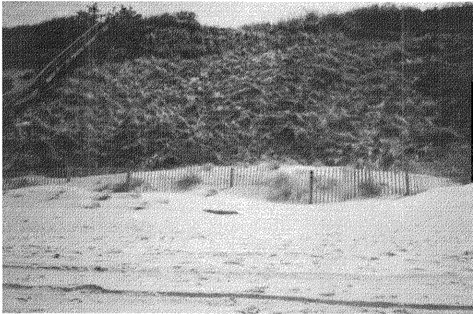
Fig 29. Completed bank stabilization project
